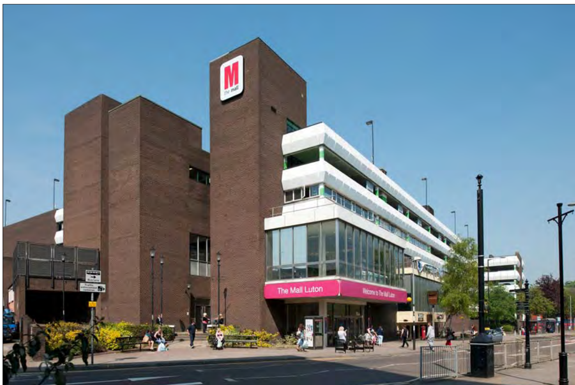
Figure 85. The eastern approach to the Arndale, Luton.
