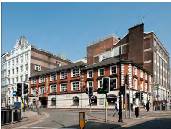
Figure 36. The easyHotel. © English Heritage NMR DPI41936.
