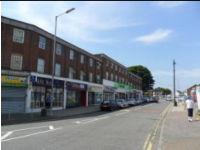
View looking north along Hitchin Road
