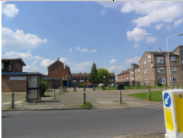
View looking north at Farley Centre
