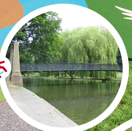
Wardown Lake suspension bridge
