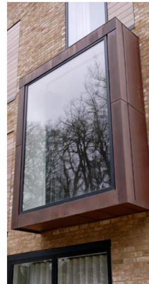
Contemporary bay windows can help to achieve required daylight conditions in rooms and add interest to the facade
