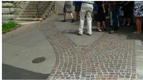
Drainage channel shall add interest to the shared surface
