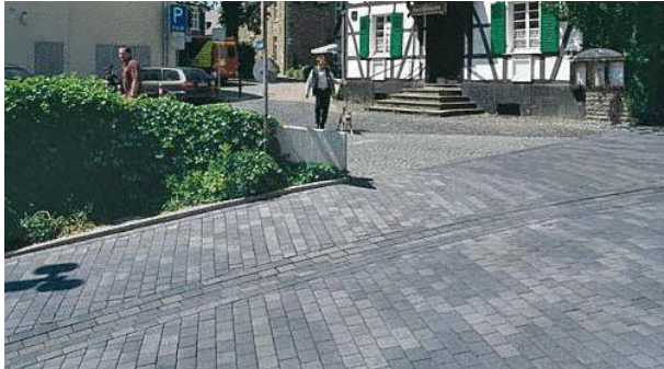
Shared space with dished drainage channel
