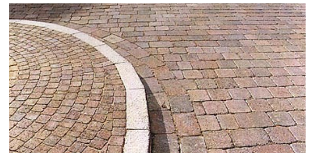
Kerb, colour contrast, change in sett size and paving pattern to mark the change in character
