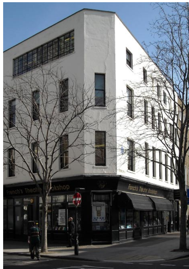
Mixed-use corner building with chamfered corner
