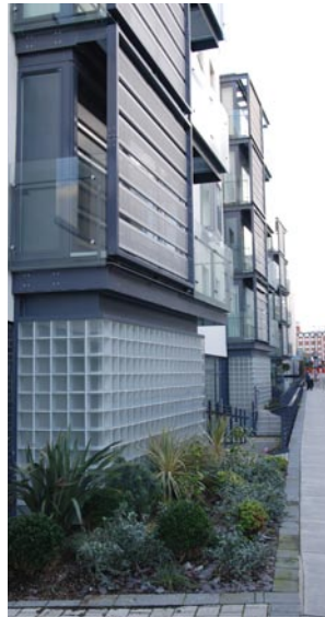
Projections can have a range of designs linking ground floor and upper floors
