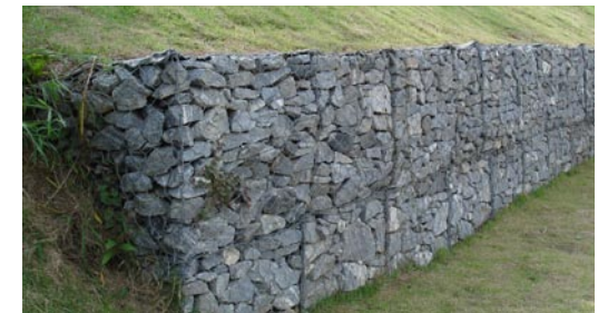
Gabions filled with recycled building material
