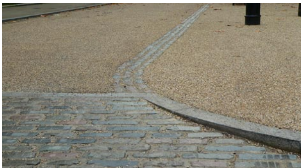
Ramp negotiates level difference and kerb height
