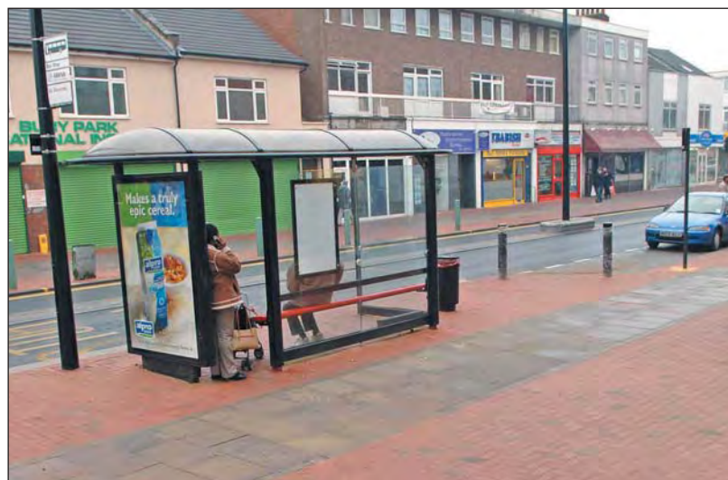
Newly installed bus shelter on Dunstable Road
