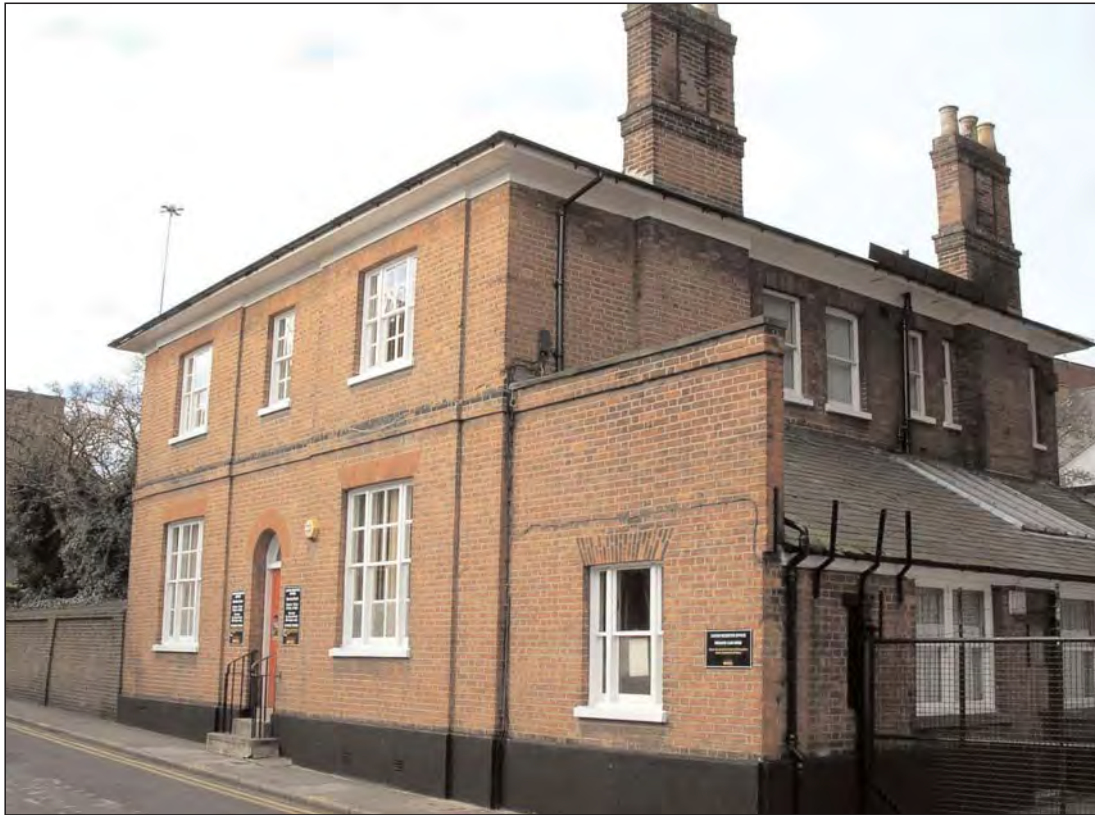
Example of a good quality Victorian building in Luton town centre conservation area
