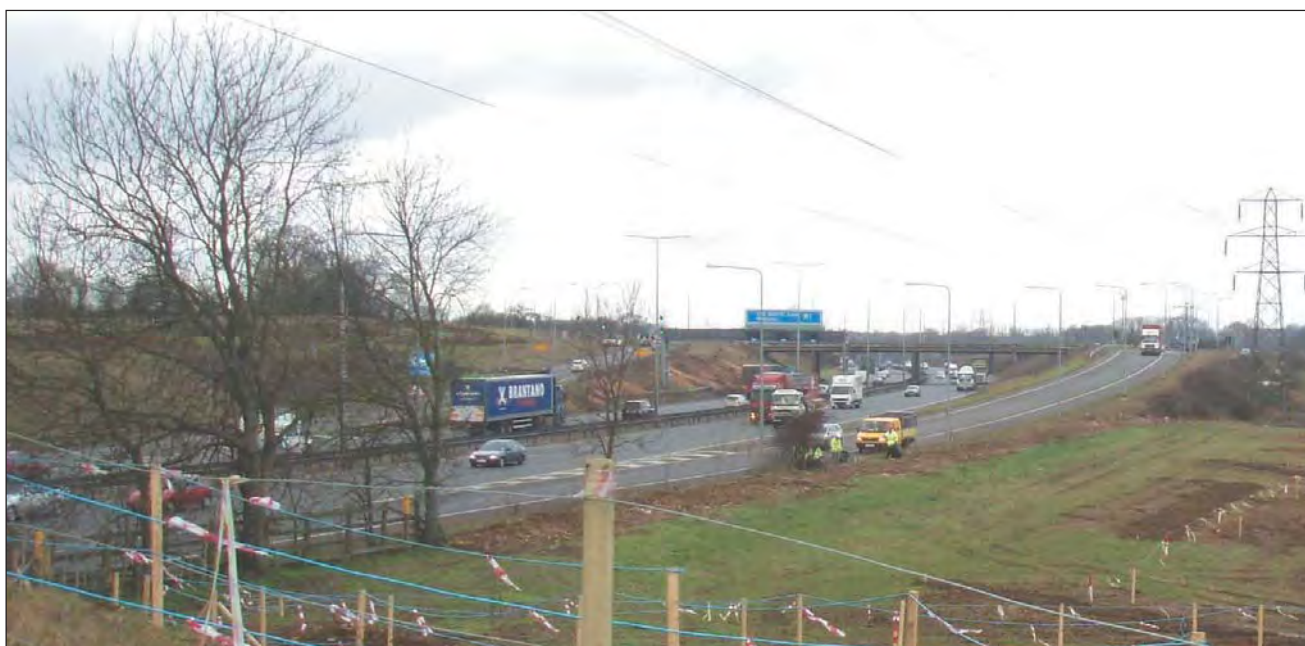
Widening of the M1 south of junction 10 commenced in 2006
