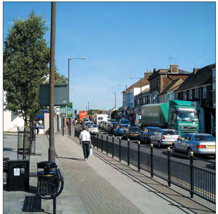
Junction of A5 and A505, which is at the centre of the Dunstable AQMA
