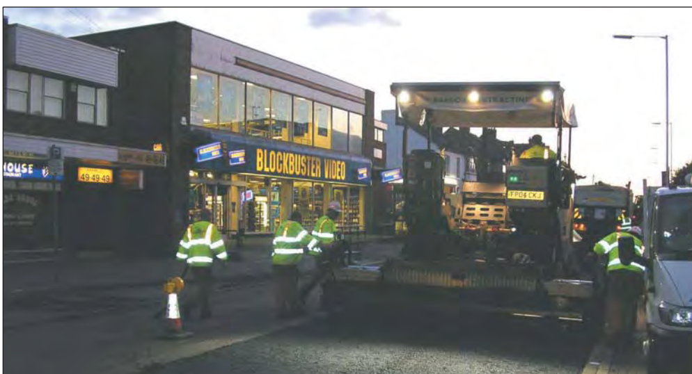
Resurfacing of the traffic-sensitive Dunstable Road during off-peak hours
