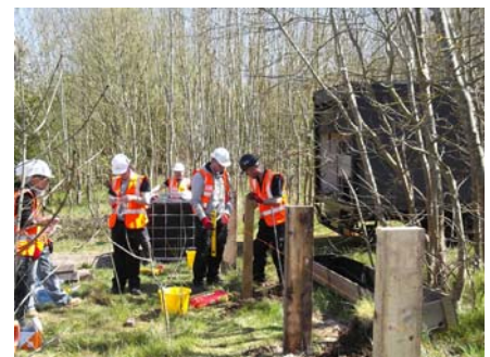
Building the fence at Henge Farm
