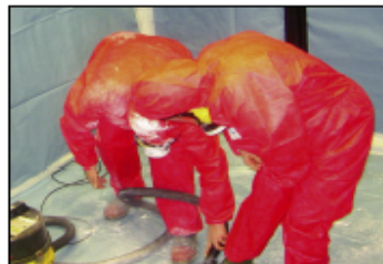
'Buddy' cleaning using a Class H vacuum cleaner
