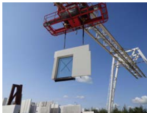
Fig. 1.10.1 Prefabricated, pre-cast concrete panels with factory fitted windows illustrate modern methods of construction on a housing project
