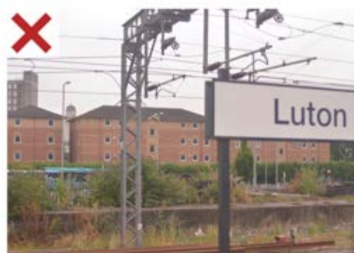
Fig. 2.2.1 Highly visible backs facing railway line
