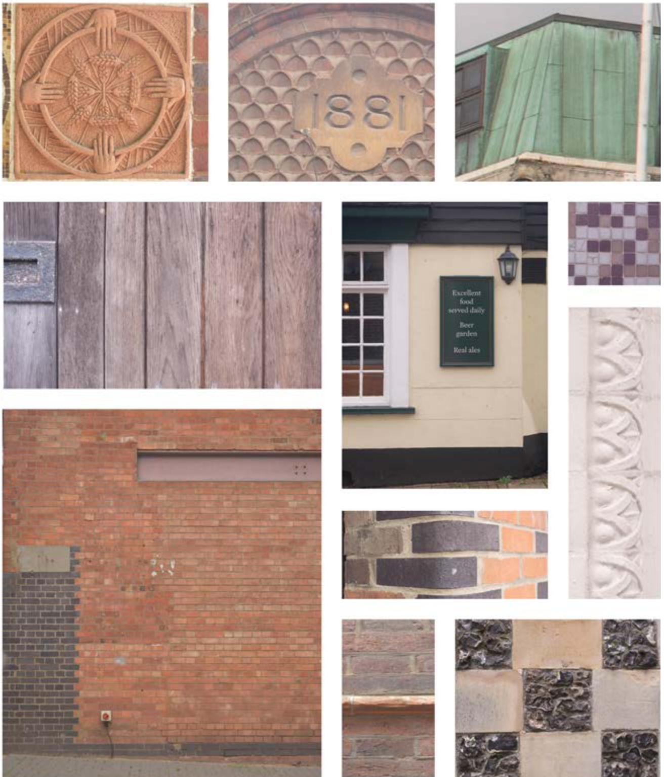
Fig. 3.5.3 High quality materials and craftsmanship evident in the town centre
