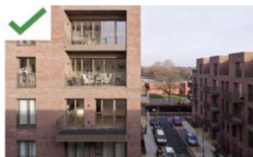
Fig. 4.3.4 Well proportioned and designed balcony spaces
