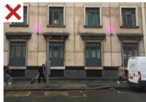
Fig. 4.7.3 External lighting should be integrated with the design of the facade rather than attached as an afterthought
