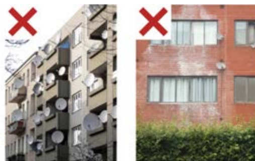
Fig. 3.2.5 Avoid cluttered façades
