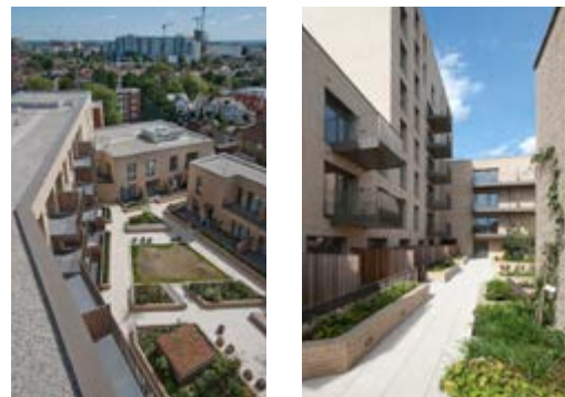
Fig. 2.12.2 Existing cross-block pathways are an important part of Luton's movement network and new attractive connections should be encouraged as part of developments
