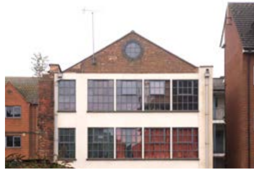
Fig. 3.3.1 Distinctive industrial roof line
