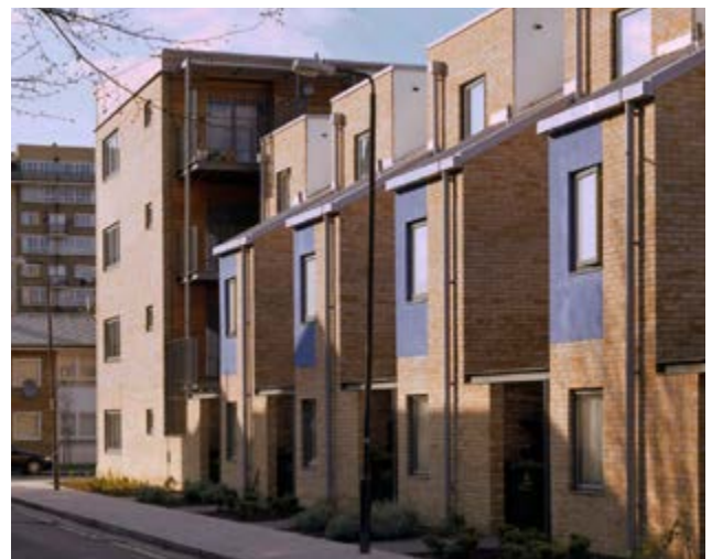
Fig. 3.4.14 Coopers Road, Southwark (ECD Architects)
