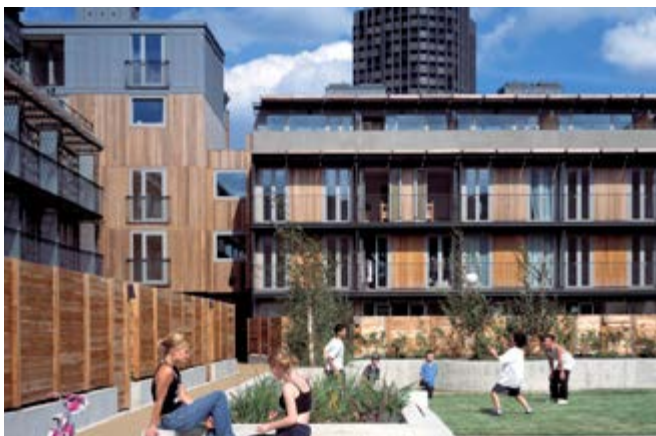
Fig. 3.2.3 Coin Street Housing, London (Community Led Housing)
