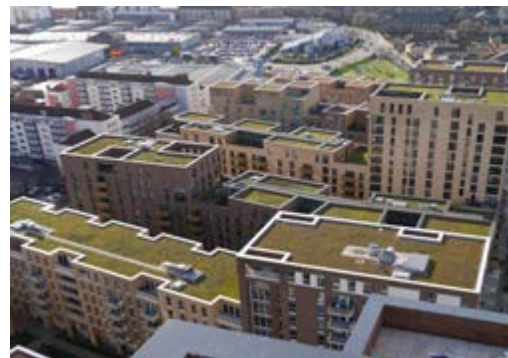
Fig. 3.3.2 Green roofs help to reduce heat-island effect
