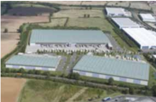
Prologis Apex Park, Daventry, Phase III
