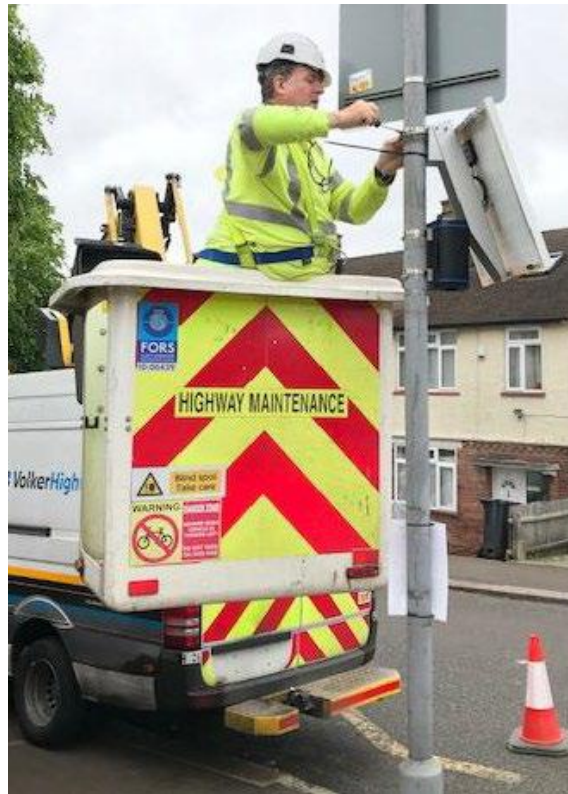
Figure 1 - Air quality sensor being installed outside Hillborough Junior School
